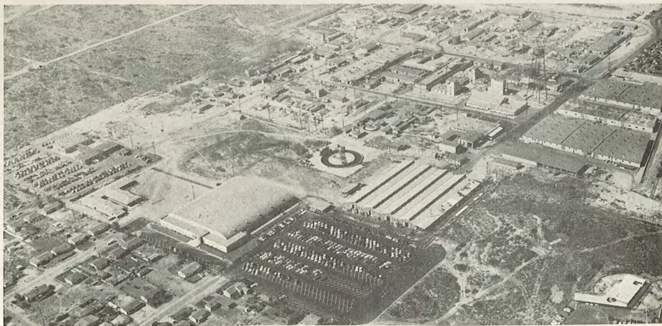
Aerojet-General's plant in Azusa, California. (Aerojet-General photo)
