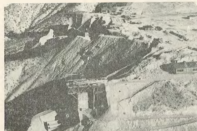
An aerial view of the Aerojet-designed rocket test stands at Edwards A.F.B. in California. — (Aerojet-General photo)
